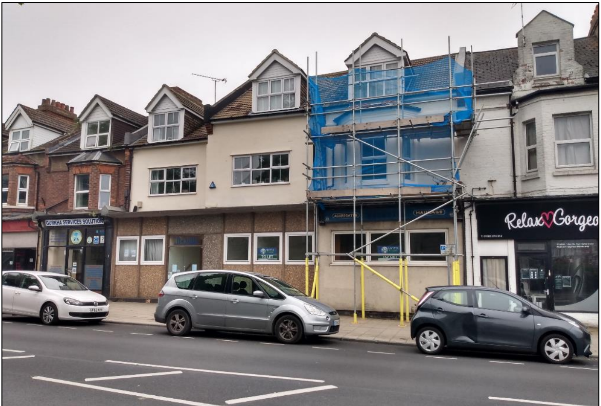
Fig.1 – Application property (to left of scaffold)
